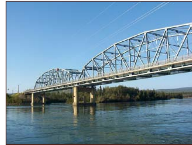
Bridge at Carmacks.
